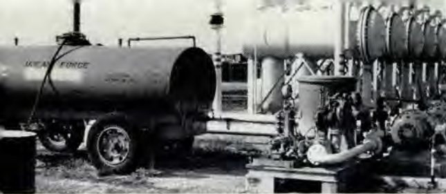
This equipment is used to inject anti-icing additive into jet fuel at WP-AFB.
